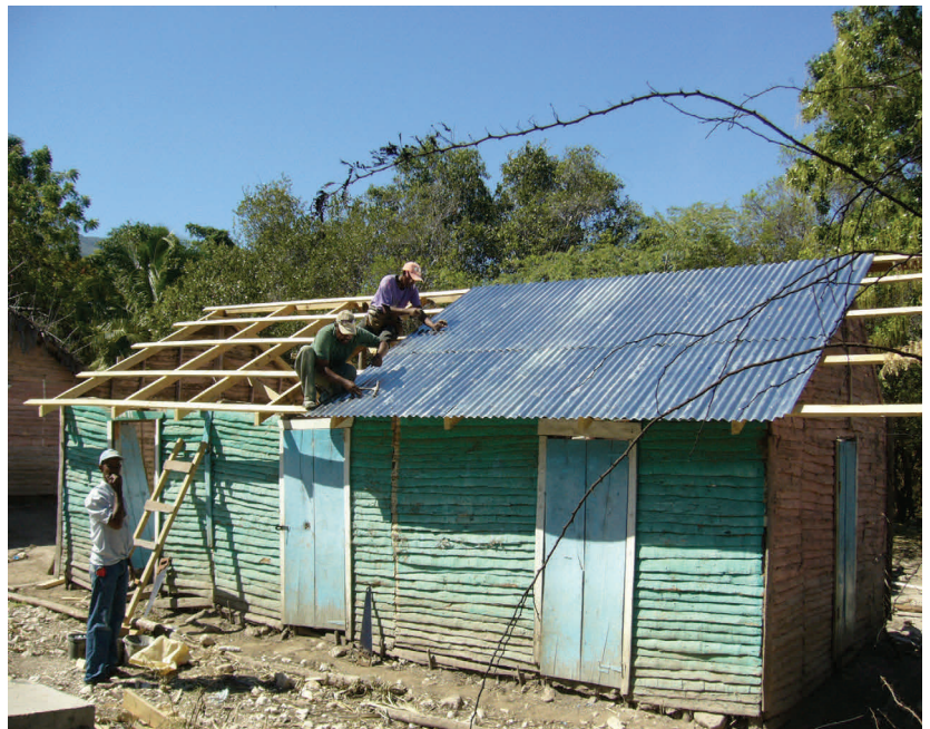
A home getting a corrugated steel roof.
