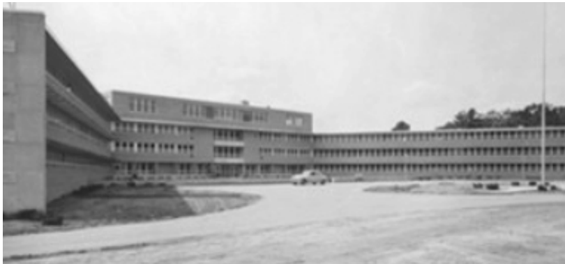
Wide view of entire east side of Heiss Hall construction
