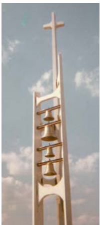
Installation of the Seminary Bells, September 1963.
